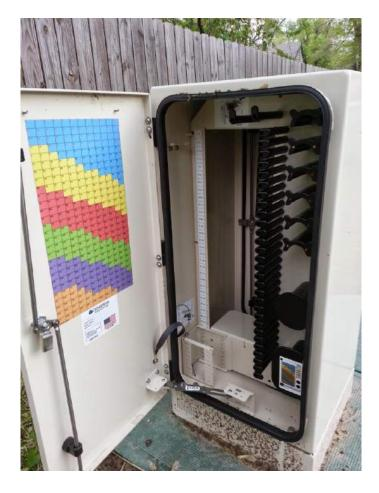
More typically, smaller PON cabinets are used, as shown in the following picture. Distributing multiple smaller cabinets maximizes the savings on fiber construction. These cabinets can be placed on the ground, as shown, but also can be mounted on poles where there is aerial fiber.
